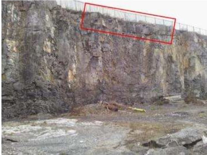
Figure 5.2: Wedge failure in the upper bench
