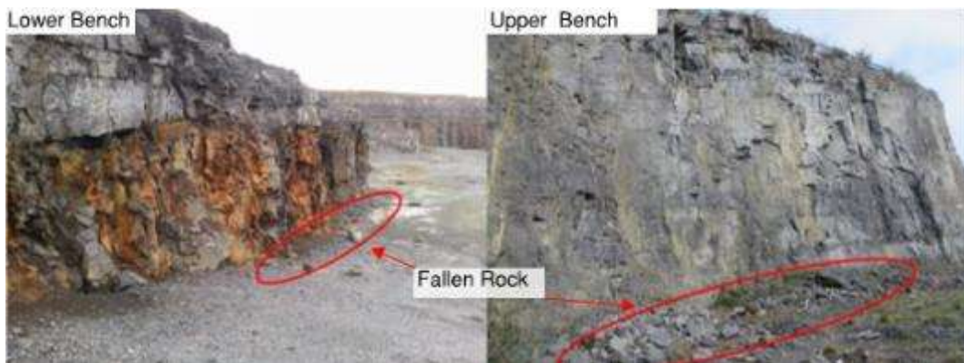
Figure 3.5: Face instability on the lower and upper bench
